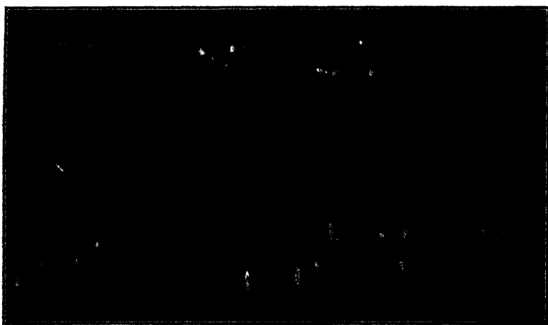
FIG. 67.—Corona on a No. 3/0 line cable. Wet.
